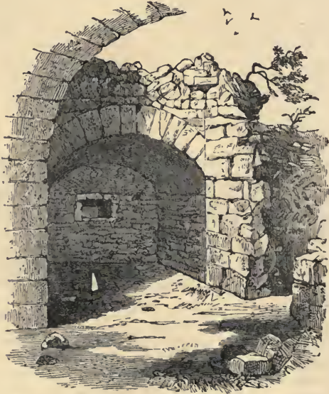
Vault where the unhappy De Ramus—the "Last of the Templars"—was buried.
